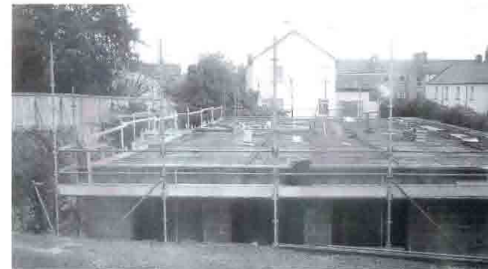
Work in progress on new Orchard Centre
