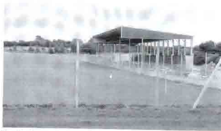
Stand under construction in September 2004
