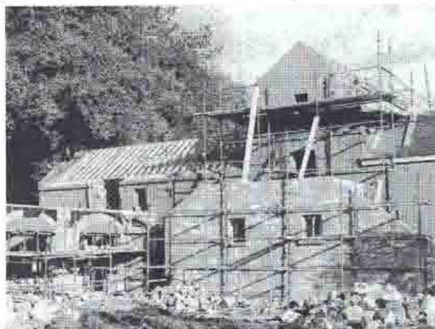
Work in progress on the new Interpretive Centre last autumn.
