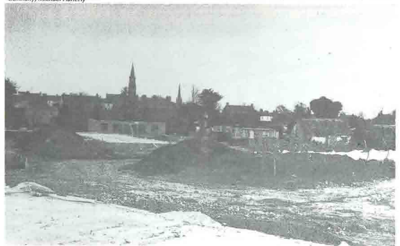
General view of construction site of new houses at Crowe Street, Gort.
