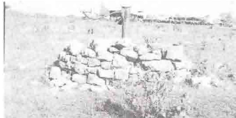
The forgotten water pump at Kinincha
