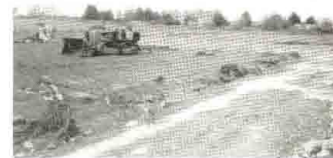
Preparing the site for a new Boy's N.S. at Tubber Road
