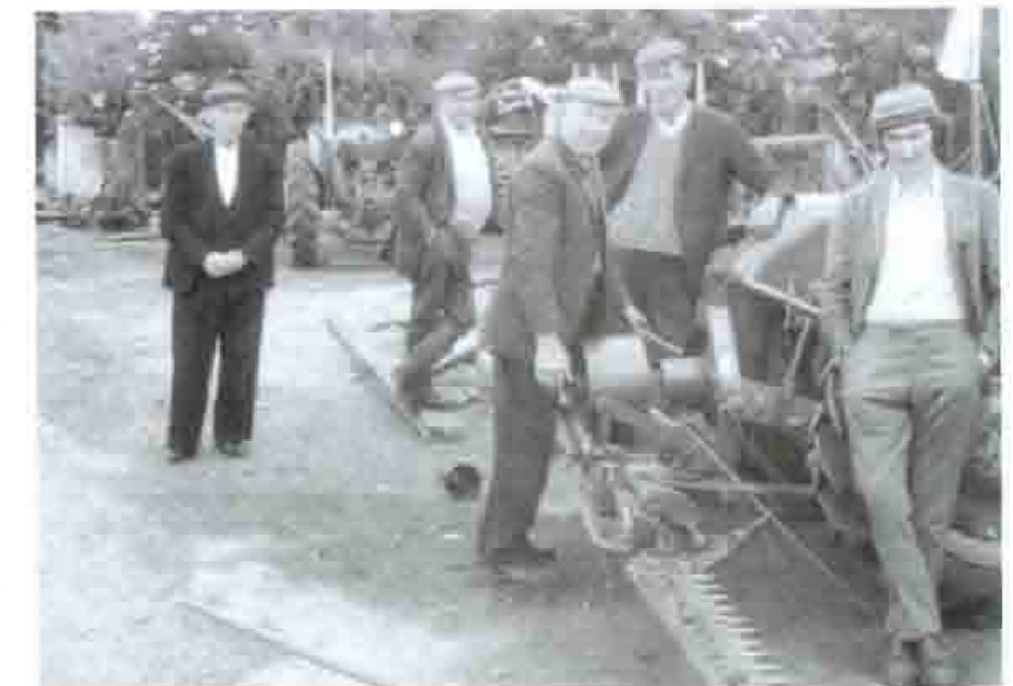
The arrival of modern machinery left to right: unknown, Bobby Hynes, Paddy Fogarty, Jimmy Nolan and Packie Byrne
